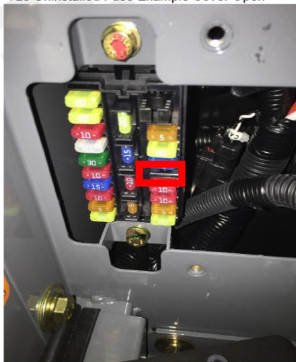
TL8 Uninstalled Fuse Example Cover Open
