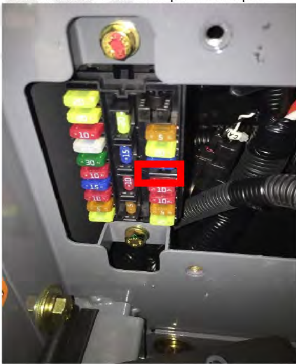
TL8 Uninstalled Fuse Example Cover Open
